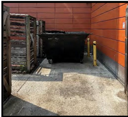
Figure 23: Above graphic depicts adequate screening for commercial dumpsters with >7-foot-high opaque fence
