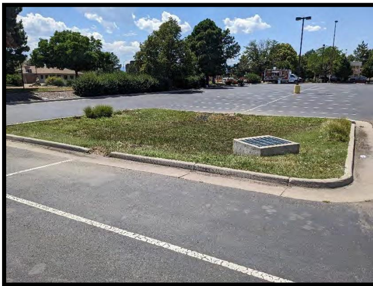
Figure 17: Above graphic describes adequate set-up for excess stormwater drainage in parking lot
