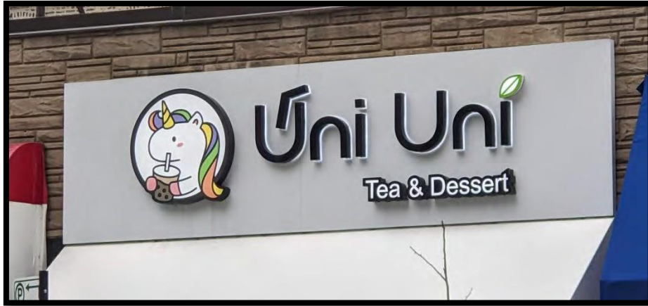
Figure 25: An image of a sign with halo-letter illumination. Uni Uni has light shining towards the gray sign background, creating the effect of a white halo around the dark, silhouetted letters.
