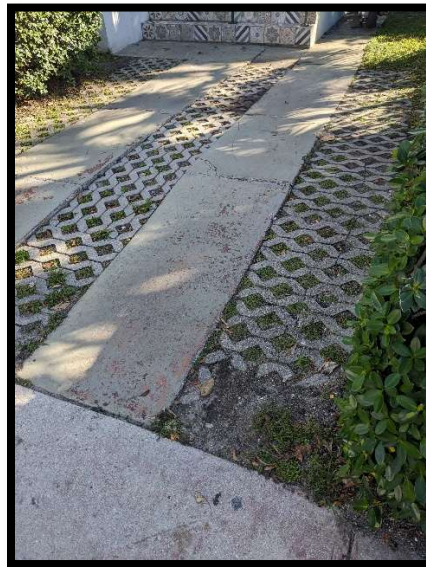
Figure 18: Graphic above describes permeable pavement used on single family parcel
