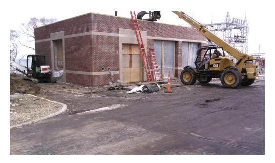
The City of Elyria Water Pumping Plant is constructing a 4.6 million dollar sludge project. It includes a 250,000 gallon sludge holding and dewatering tank and centrifuge to remove solids from the sludge. Sludge at 2-4% solids enter the centrifuge where it is the sludge is spun and the solids are separated from the water. Solids are then dumped into a trailer for disposal in local landfill facilities.
