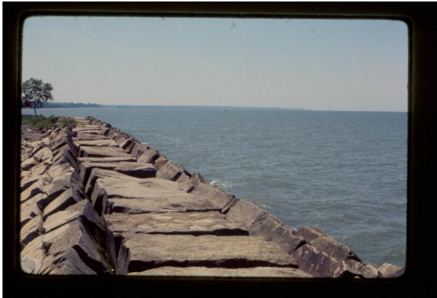
Water Plant break wall to Lake Erie
