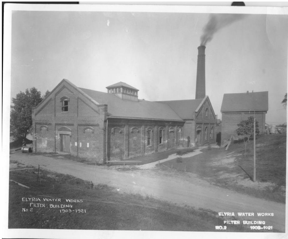
Original filter building built in 1903
