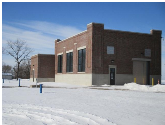
NEW HIGH SERVICE PUMP HOUSE
